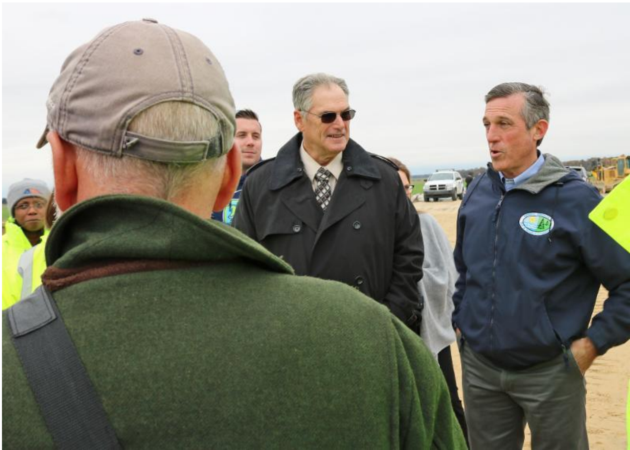
In photo, from left: State Rep. Charles Postles joined Gov. John Carney and transportation officials Tuesday morning at the construction site of the South Frederica Grade-Separated Intersection on Delaware 1.
